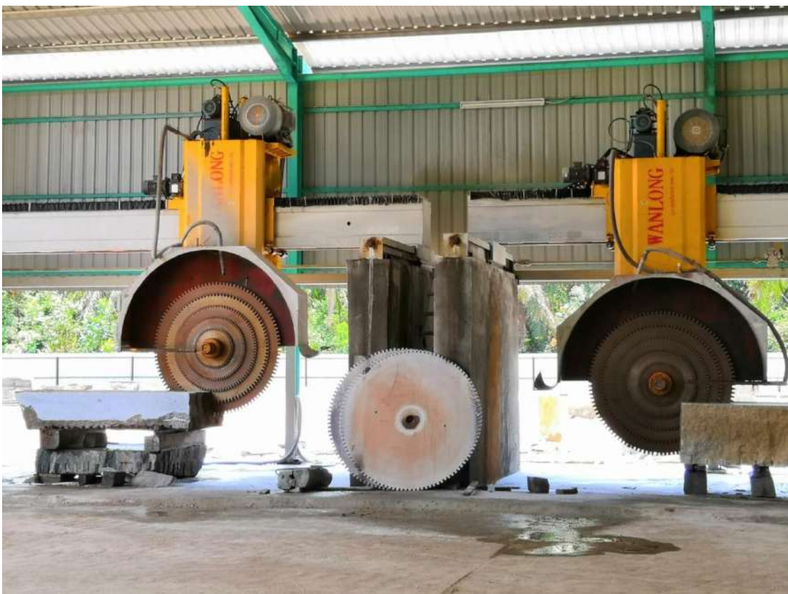
New multi-blade block cutters with more efficient operations at Bukit Chetai Granite Quarry
